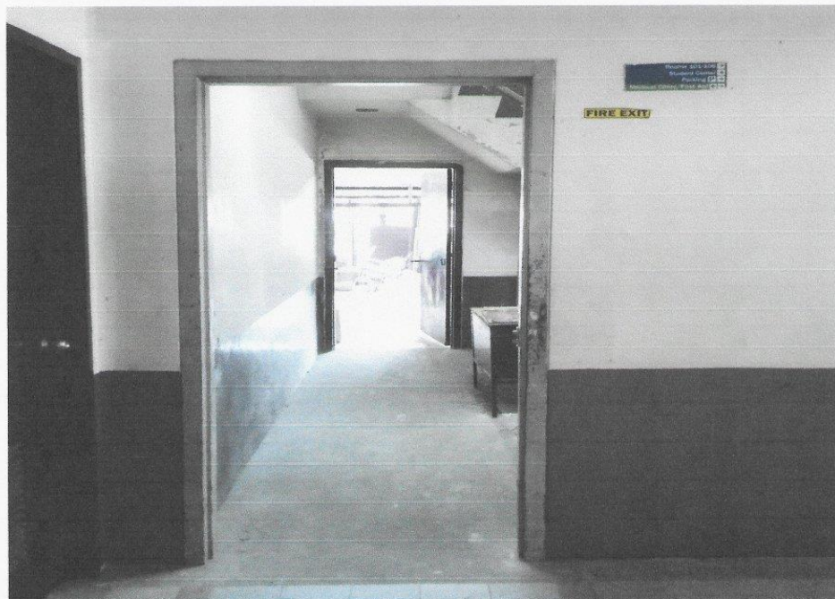
EMERGENCY EXIT SIGNAGE AT COLLEGE OF ENGINEERING AND ARCHITECTURE BUILDING
