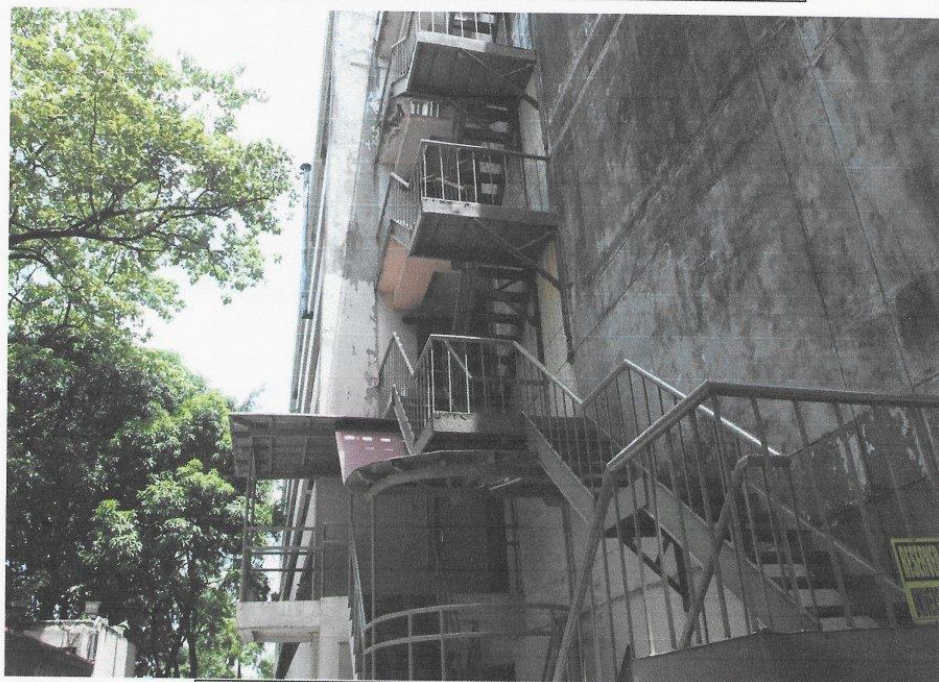
EMERGENCY EXIT AT MAIN BUILDING
